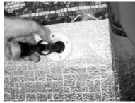
8. Make sure the rubber insert is in place before inserting the lens into the fitting.
