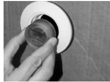
8. Install the lens assembly into the wall fitting. It may be necessary to have someone cautiously pull the cable from the other end.
