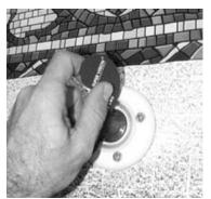
11. Tighten the retaining ring with the lens wrench until it is snug.
