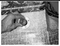
9. Install the lens assembly into the wall fitting. It may be necessary to have someone cautiously pull the cable from the other end.
