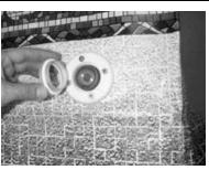
10. Place the retaining ring over the lens and turn clockwise to tighten. Make sure the two rubber gaskets are in place before you install the retaining ring.
