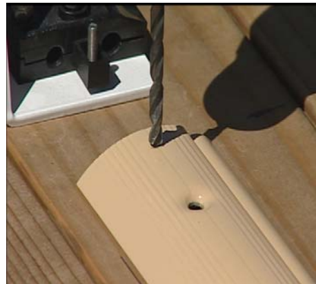
Drill a 1/4" hole into the track.
