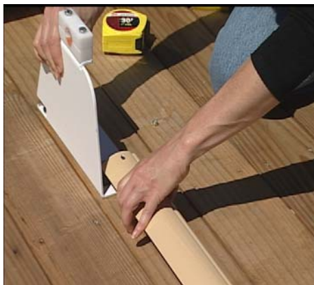
Push the track down over the stud.
