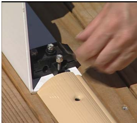
Remove the top of the track guide
